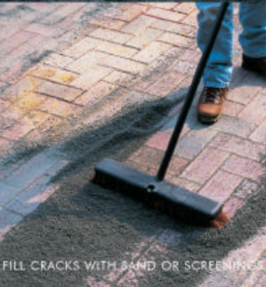
LEVEL SAND OR STONE SCREENINGS
