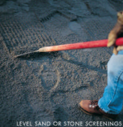
AFTER EXCAVATION, APPLY GRAVEL LAYER
